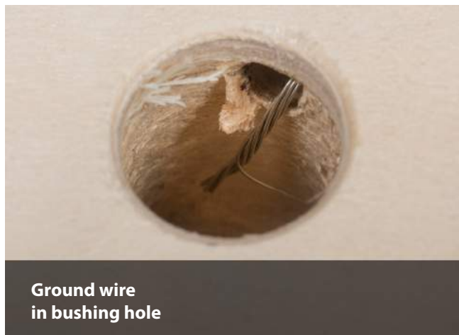
Bushing hole before chamfering
